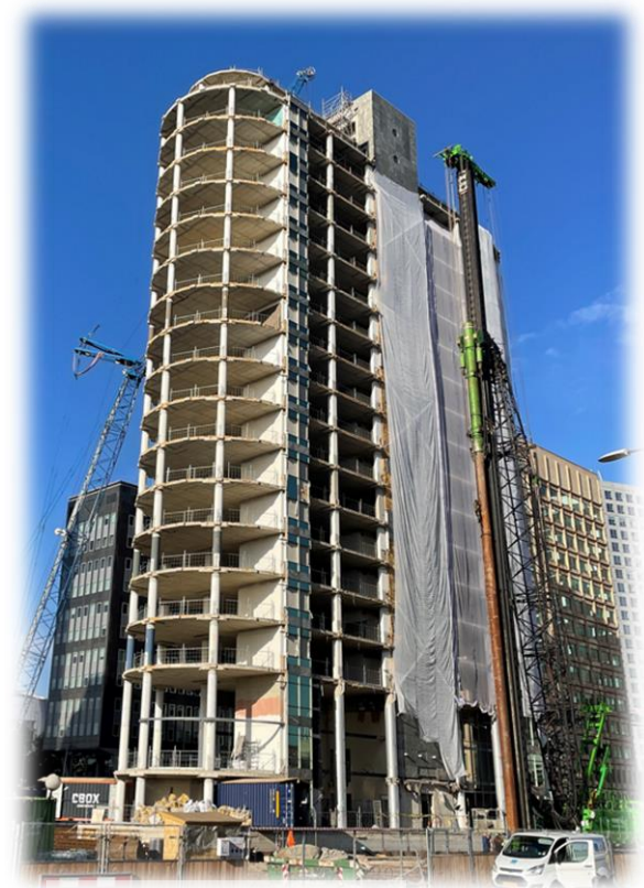
Current state of office tower
