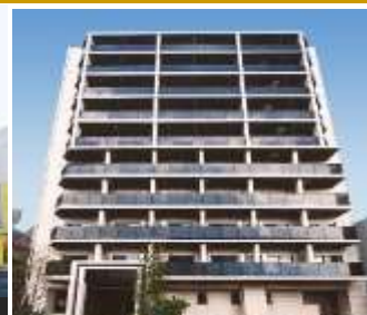
City Lux Yokohama (78 units)
