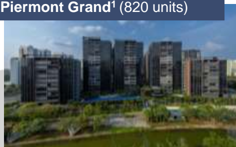
Piermont Grand 1 (820 units)
