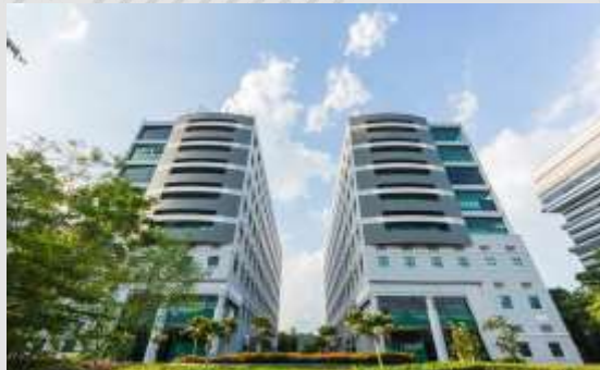
Citilink Warehouse (8 strata units)
