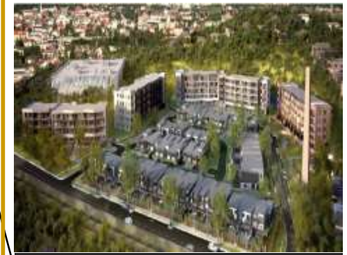
Project on Mina Parade (Residential)
