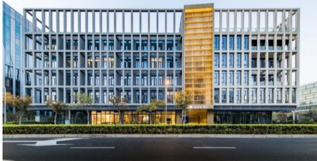
Shanghai Hongqiao Sincere Centre (Phase 2)
