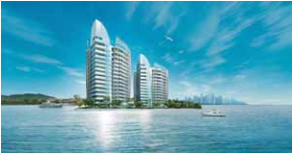
Designed for water and energy efficiency, The Oceanfront @ Sentosa Cove is the first private residential project to receive the BCA Green Mark Platinum Award.
