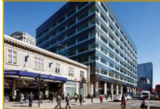
Asset Refurbishment @ Aldgate House
